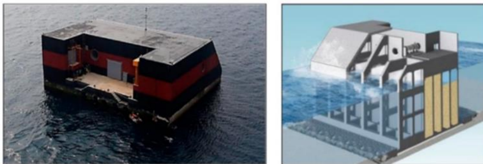
Fig. 5. Back view (left) and perspective view (right) of the OWC factory in Yongsoo [3]
