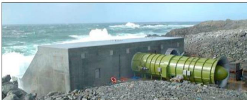
Fig. 3. LIMPET OWC plant installed on the island of Islay, Scotland [24]
